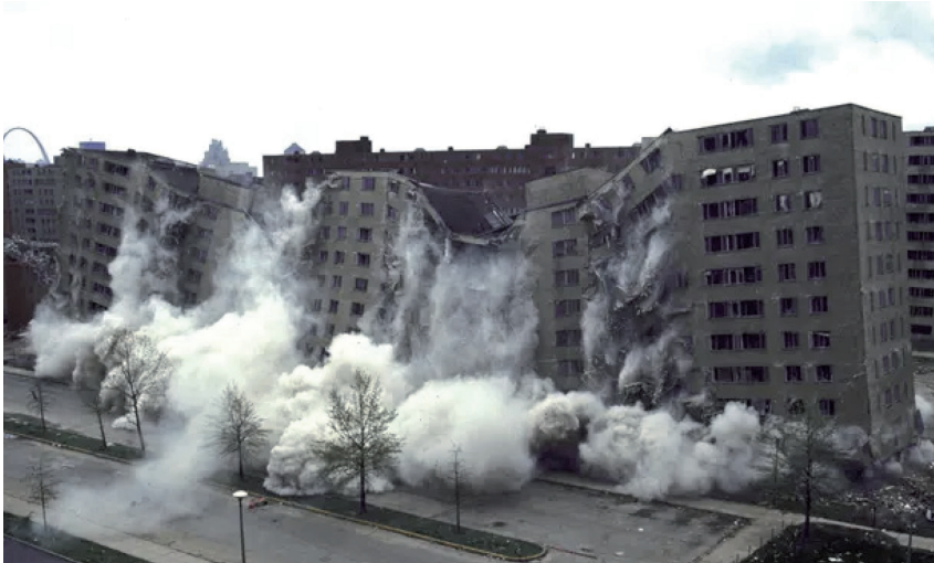
The Second Stage of Demolition of Pruitt-Igoe in April 1972 48
