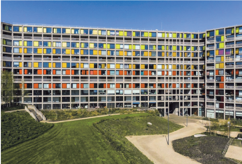
Park Hill Estates, Sheffield England, Undergoing Restoration, 2019 30
